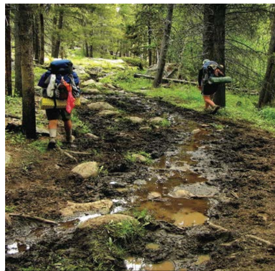
Heavy horse traffic has compacted and incised the main tread, which captures and retains water; subsequent hikers and horse riders seeking to avoid mud-holes and widen trails (Marion et al, 2016).
